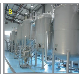
10 ton Plant scale bioreactor
